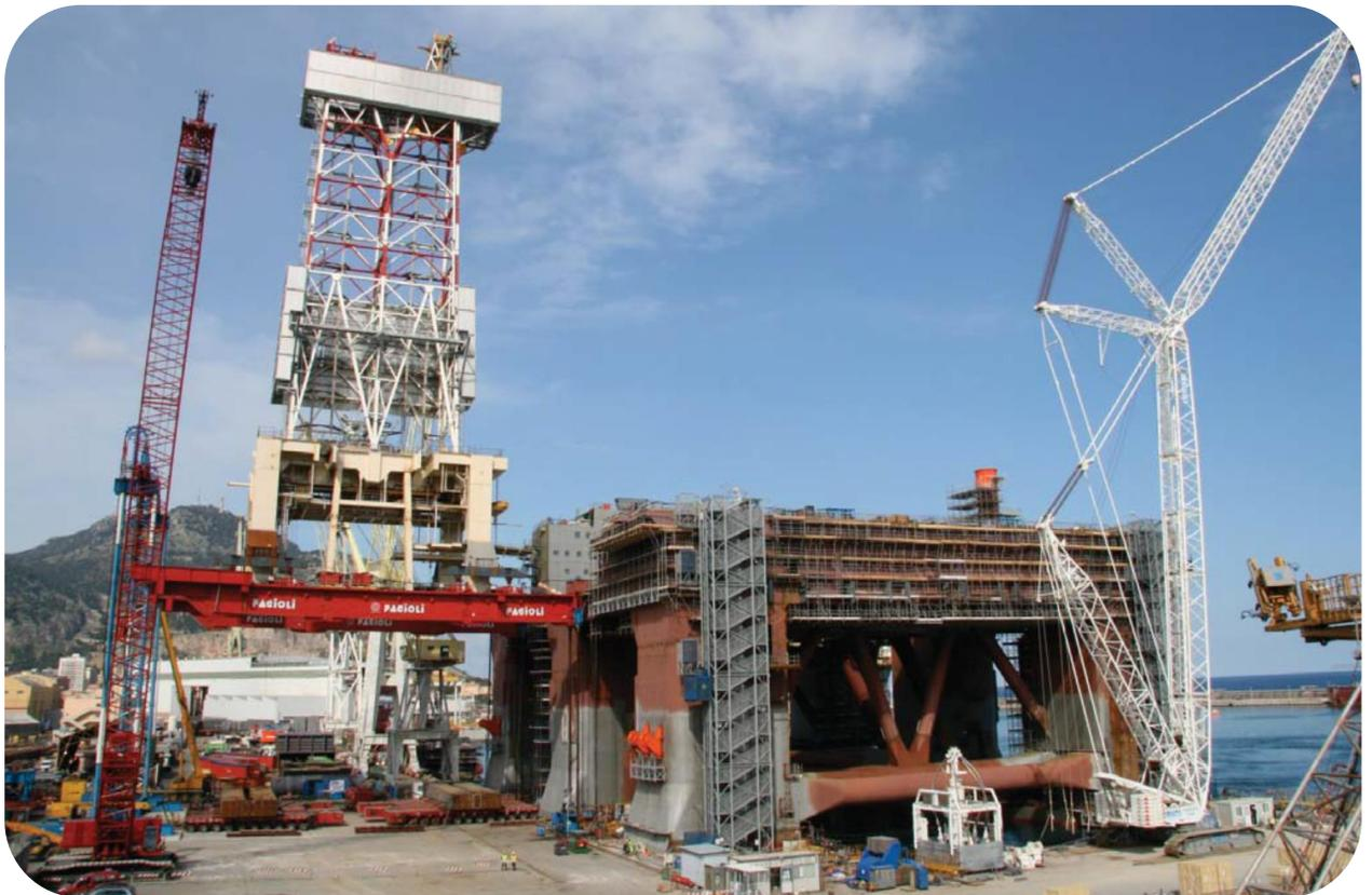
But it was the second part of the project, performed two months later that was the most extraordinary, the installation of the huge drilling rig tower which was an impressive 90m high and weighing 2,400 tonnes.
